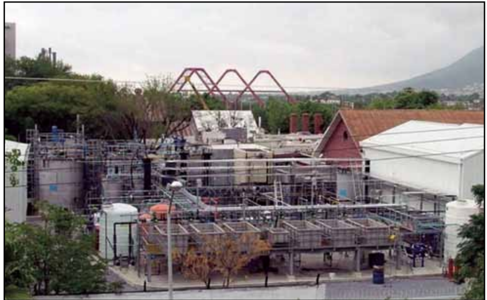
Penoles, Mexico demonstration bioleaching plant built by BacTech
